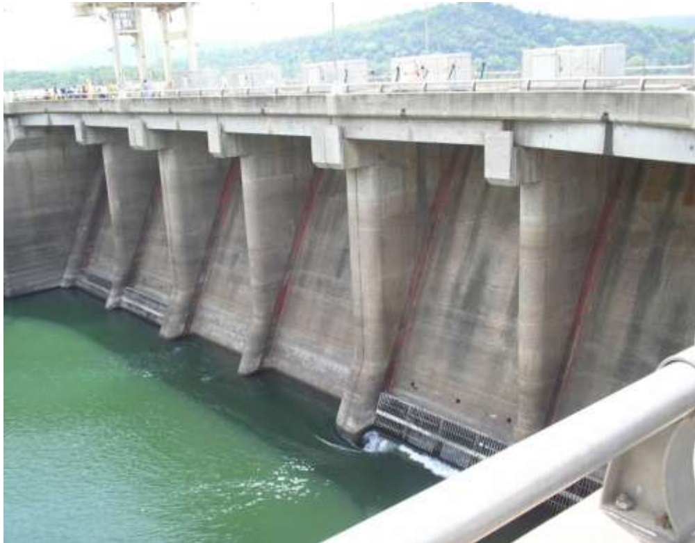
Figure 2.4 The Akosombo Dam
