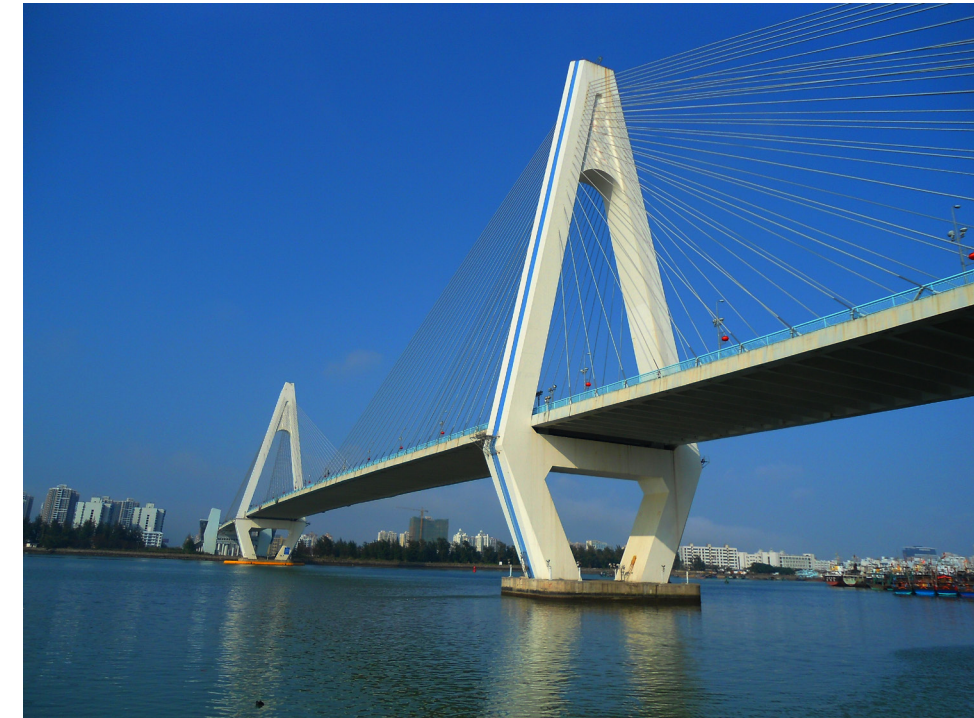
Figure 8.10: Sample bridge to be constructed along strategic locations on the Volta Lake
