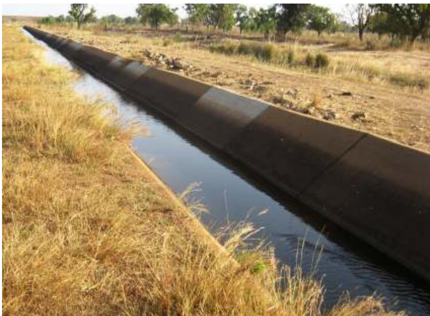
A Canal from large scale dam
