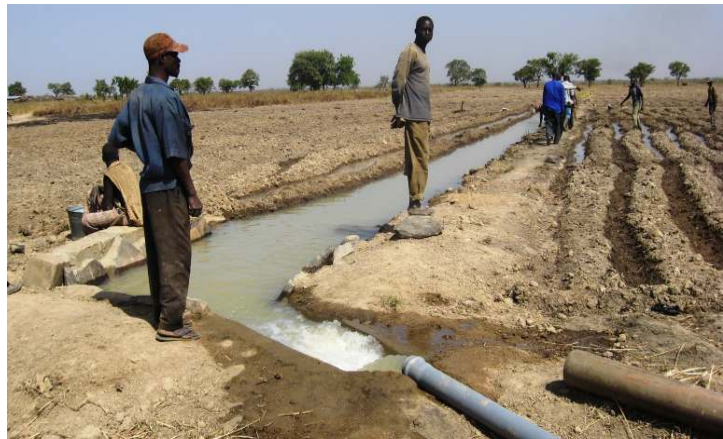
Formal Irrigation system
