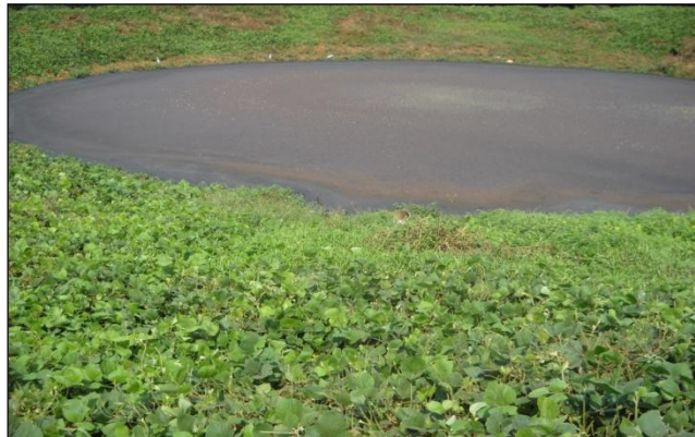
Figure 6.11: POME treatment pond
