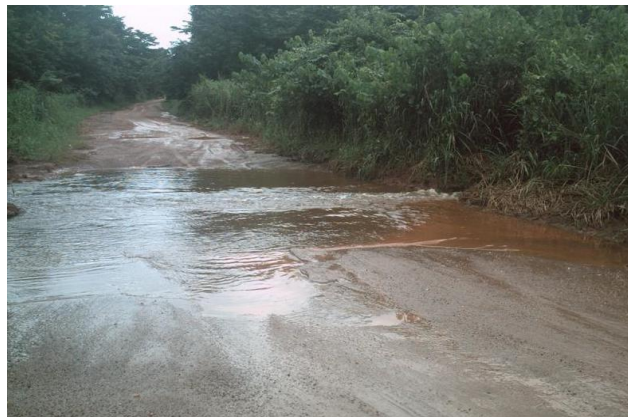
Figure 6.6: Flooded road linking an oil palm farming community to the outside world
