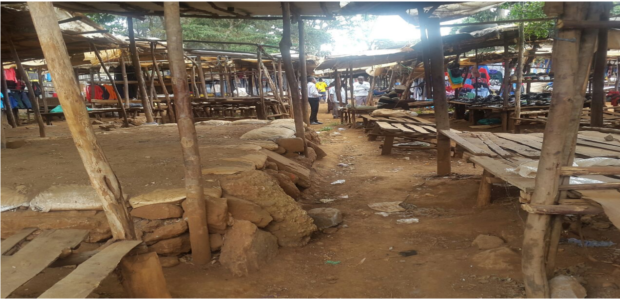
Plate 3: Temporary structures in Ruiru Market
