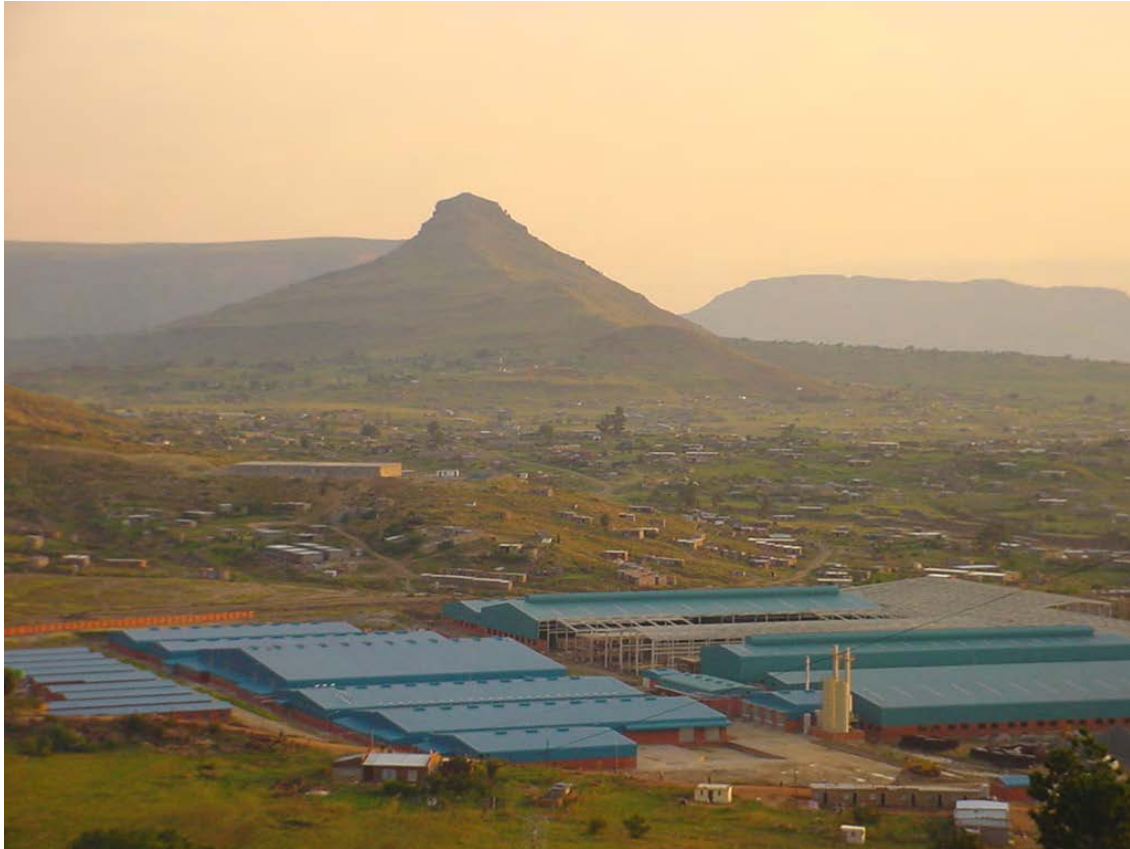
Plate 6: New Factory under construction in Maseru: AGOA has stimulated investment
