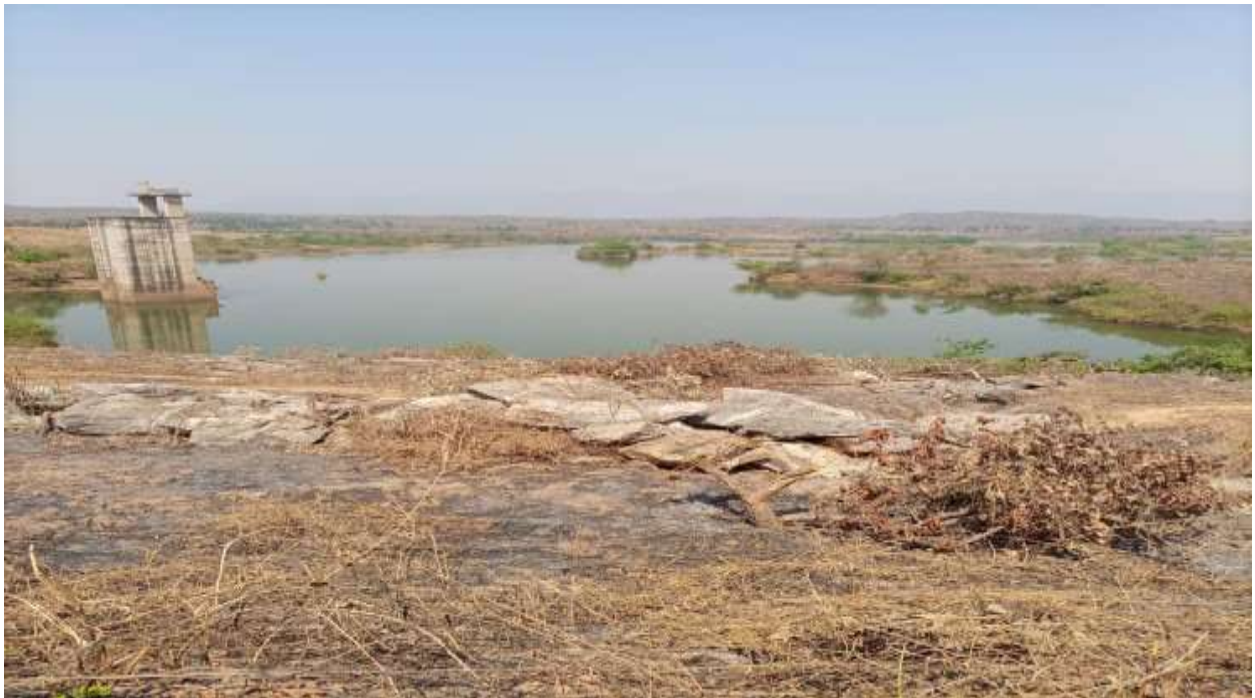
Plate 16: Farin Ruwa Dam Intake Tower
