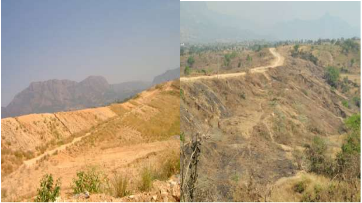
Plate 15: Farin Ruwa Dam Embankment
