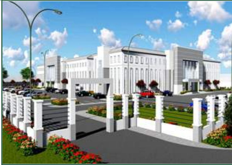
Construction of New Secretariat Office Complex
