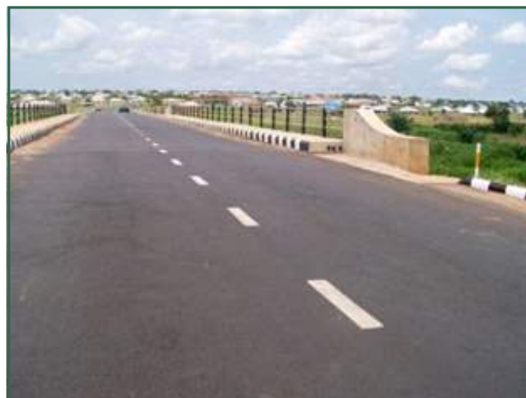
Construction of Road Projects (Zango-Akerebiata)
