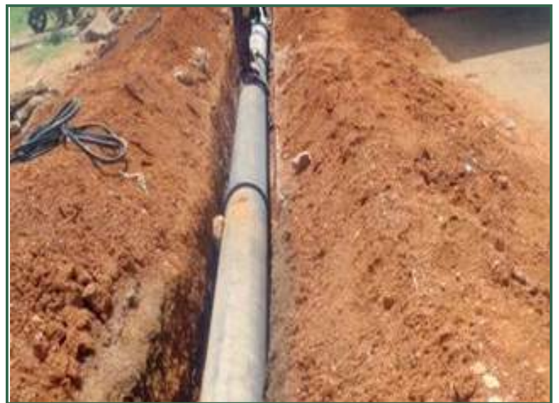
Ongoing water reticulation projects in Ilorin Metropolis
