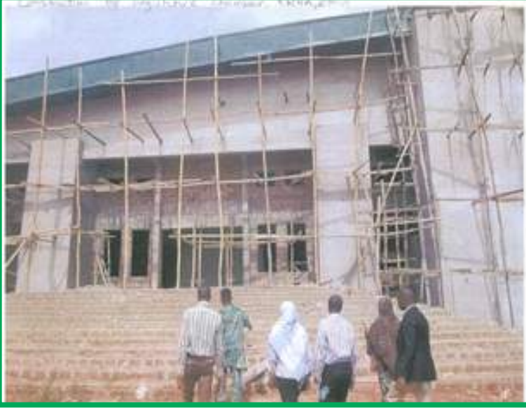
Construction of Legislative chamber, KWHA, Ilorin
