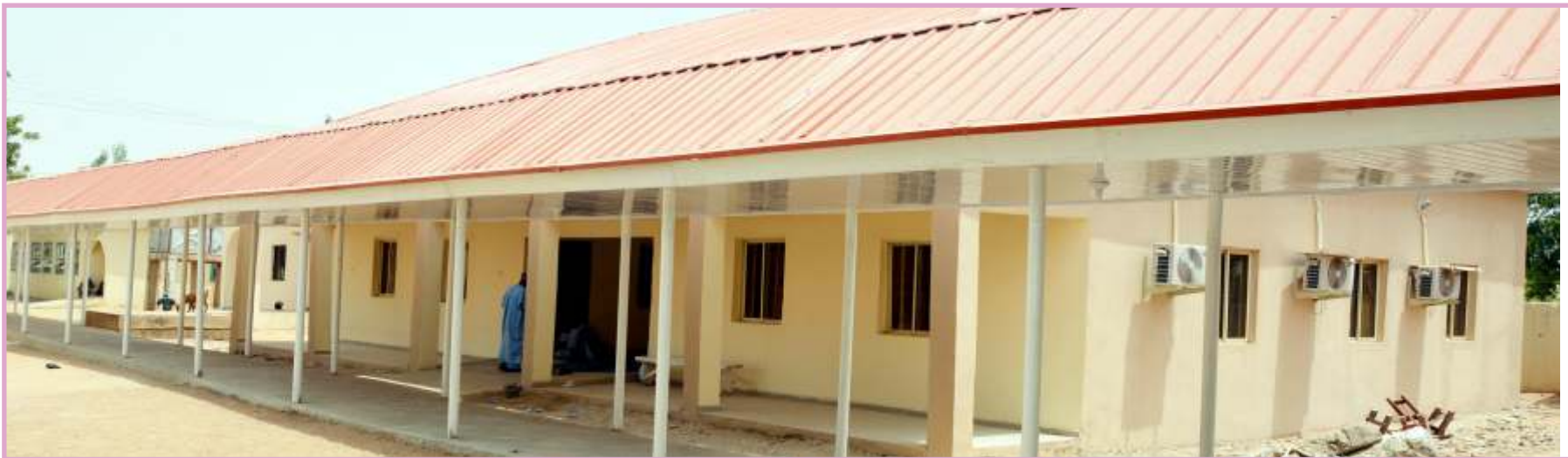
Maryam Abatcha Maternity Hospital upgraded and retrofitted by the Gaidam administration
