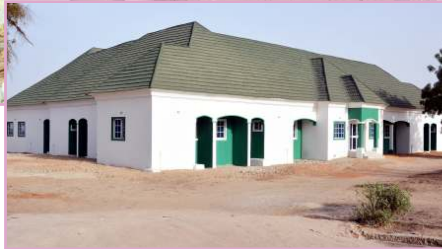
State Assembly Service Commission new office building
