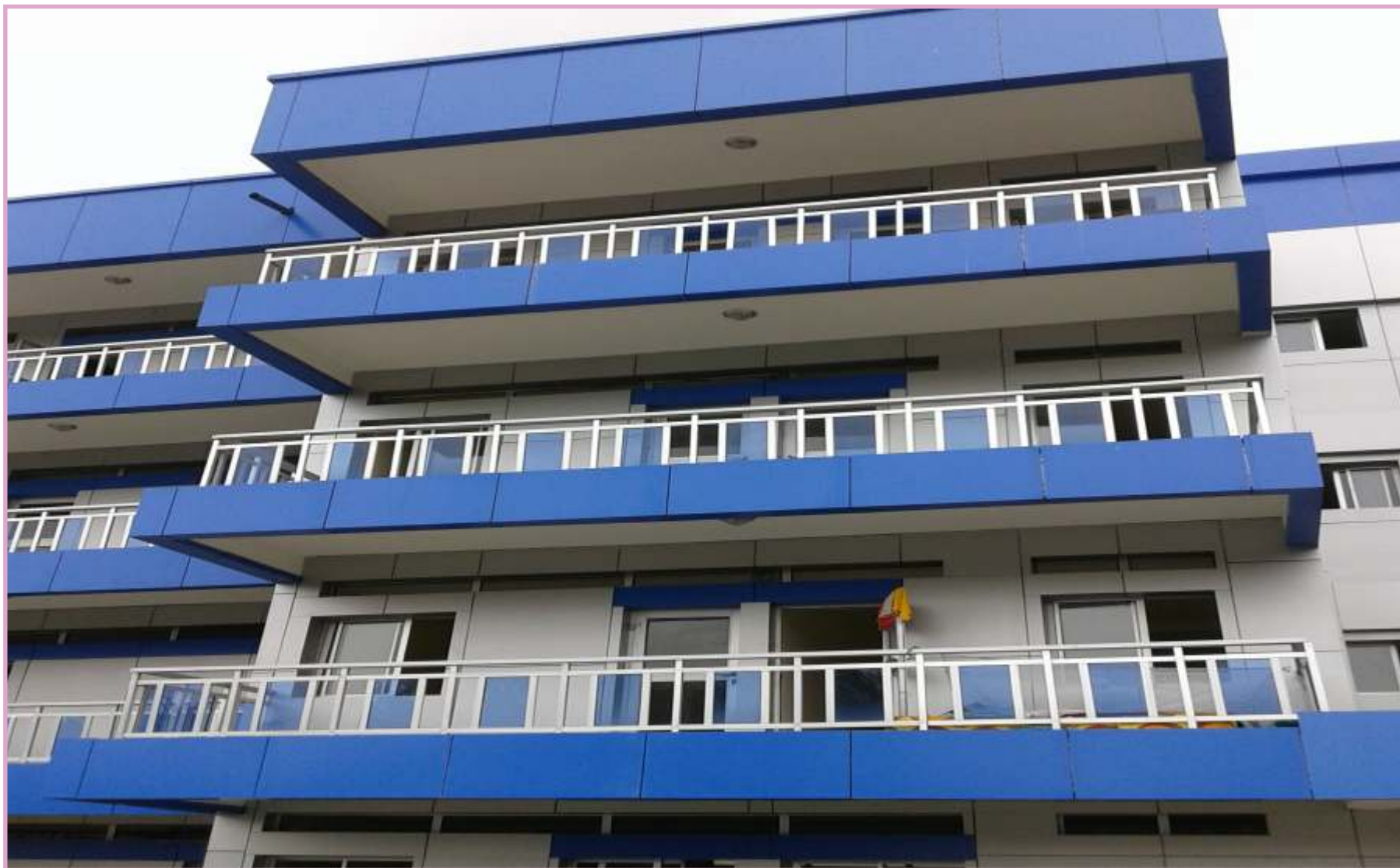
Yobe Liaison Office, Lagos renovated and upgraded by Gov. Gaidam administration
