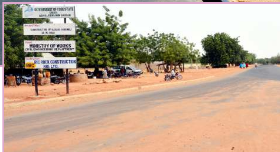
Maiduwa - Gadaka road built by the Gaidam administration
