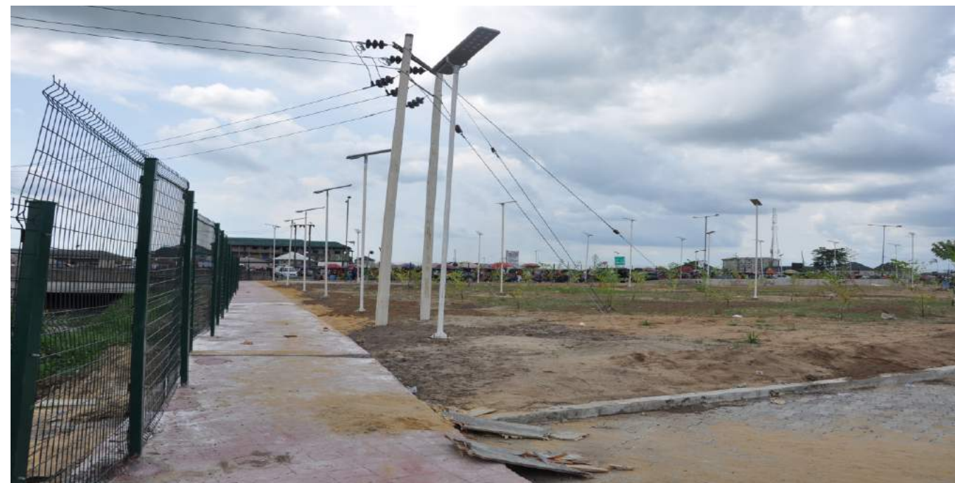
TOMBIA ROUNDABOUT EXPANSION BEAUTIFICATION ON-GOING
