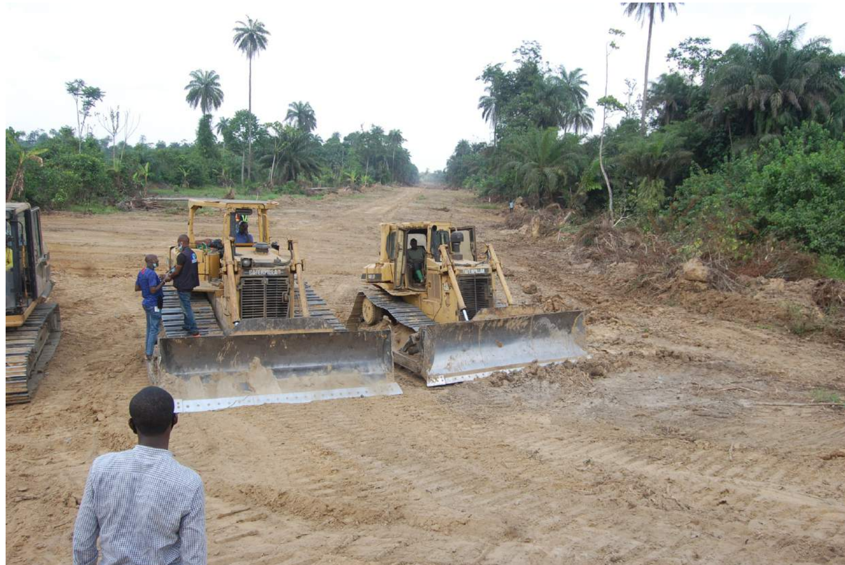
AMASSOMA IGBEDI ROAD ON-GOING
