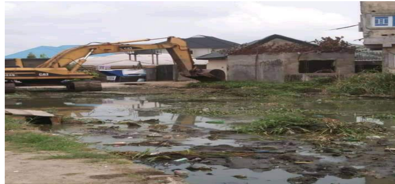
SAPTEX, OKAKA, OSIRI & PDP ROADS ON-GOING
