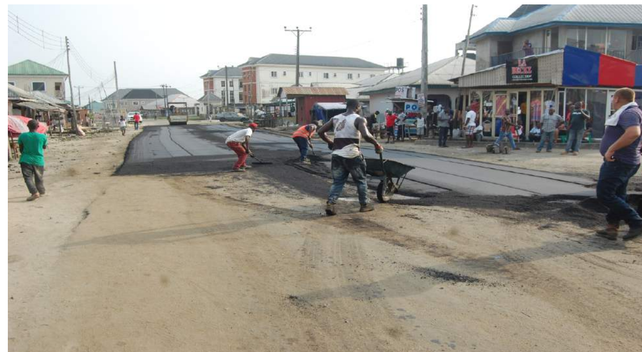
SAPTEX, OKAKA, OSIRI & PDP ROADS ON-GOING
