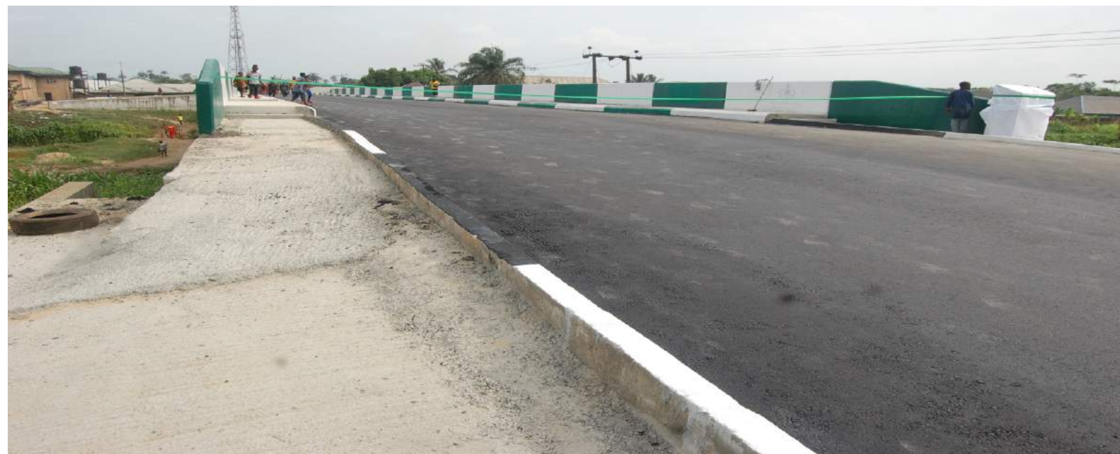
IMIRINGI BRIDGE COMPLETED
