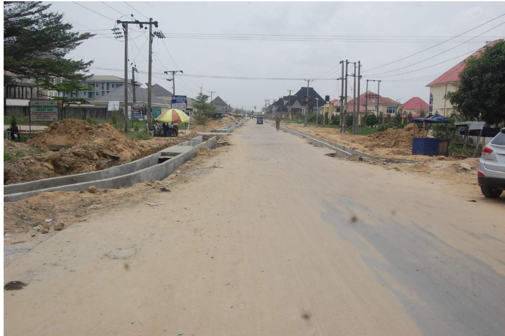
COMMISSIONERS ESTATE ROAD OPOLO ON-GOING
