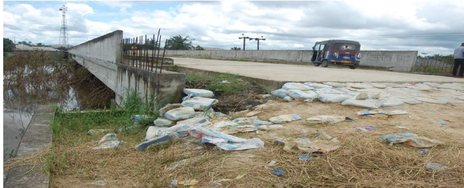
IMIRINGI BRIDGE ON-GOING
