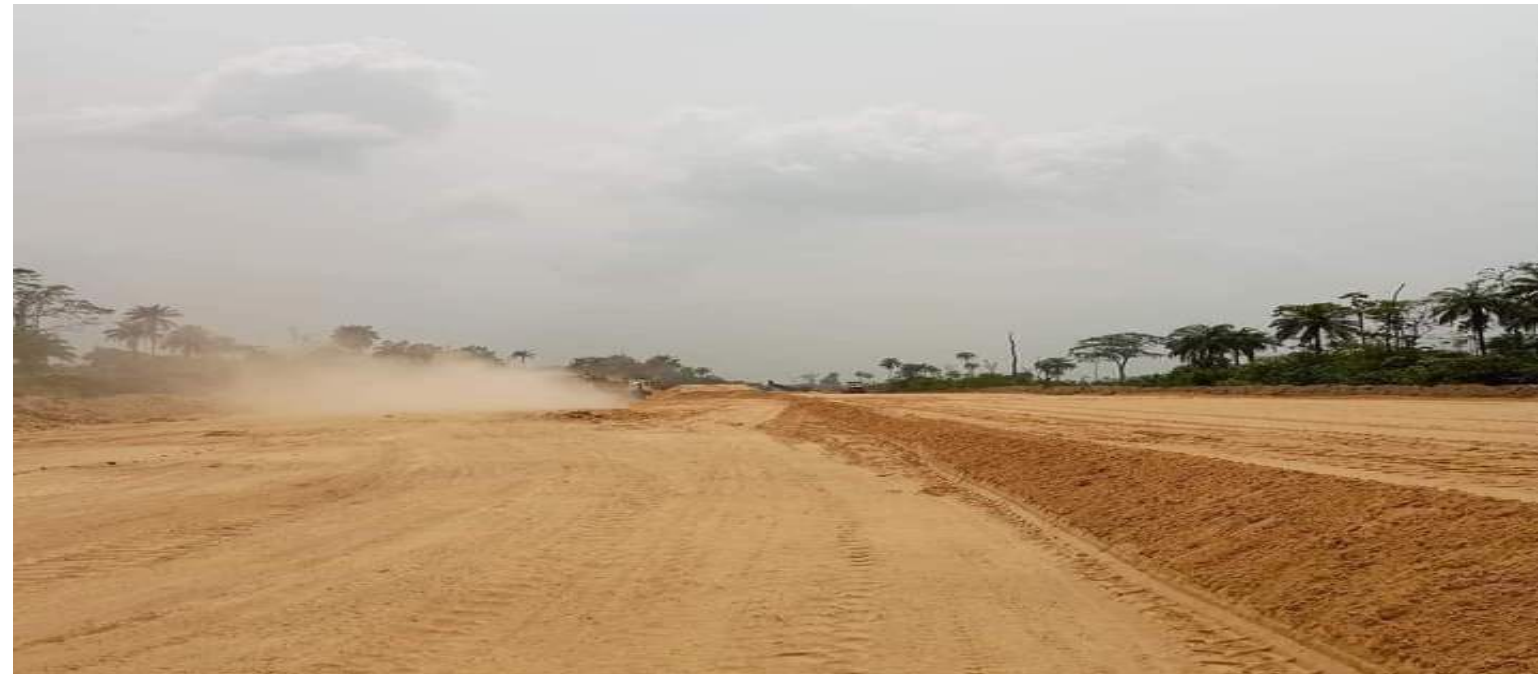
IGBOGENE AIT OUTER RING RD ON-GOING
