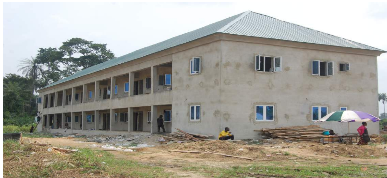
VOCATIONAL CENTRE SAMPOU ON-GOING
