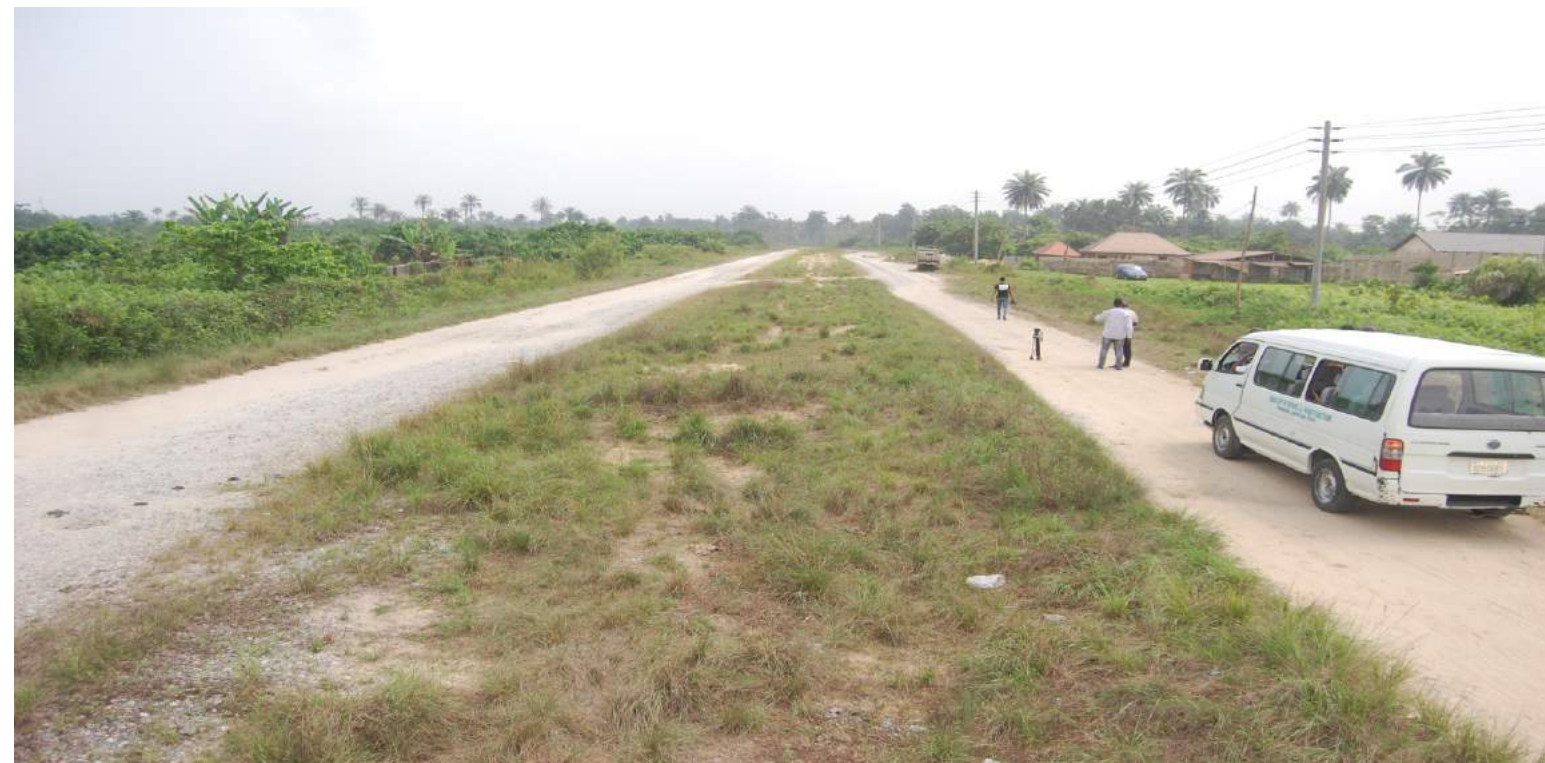
IGBOGENE AIT OUTER RING RD ON-GOING
