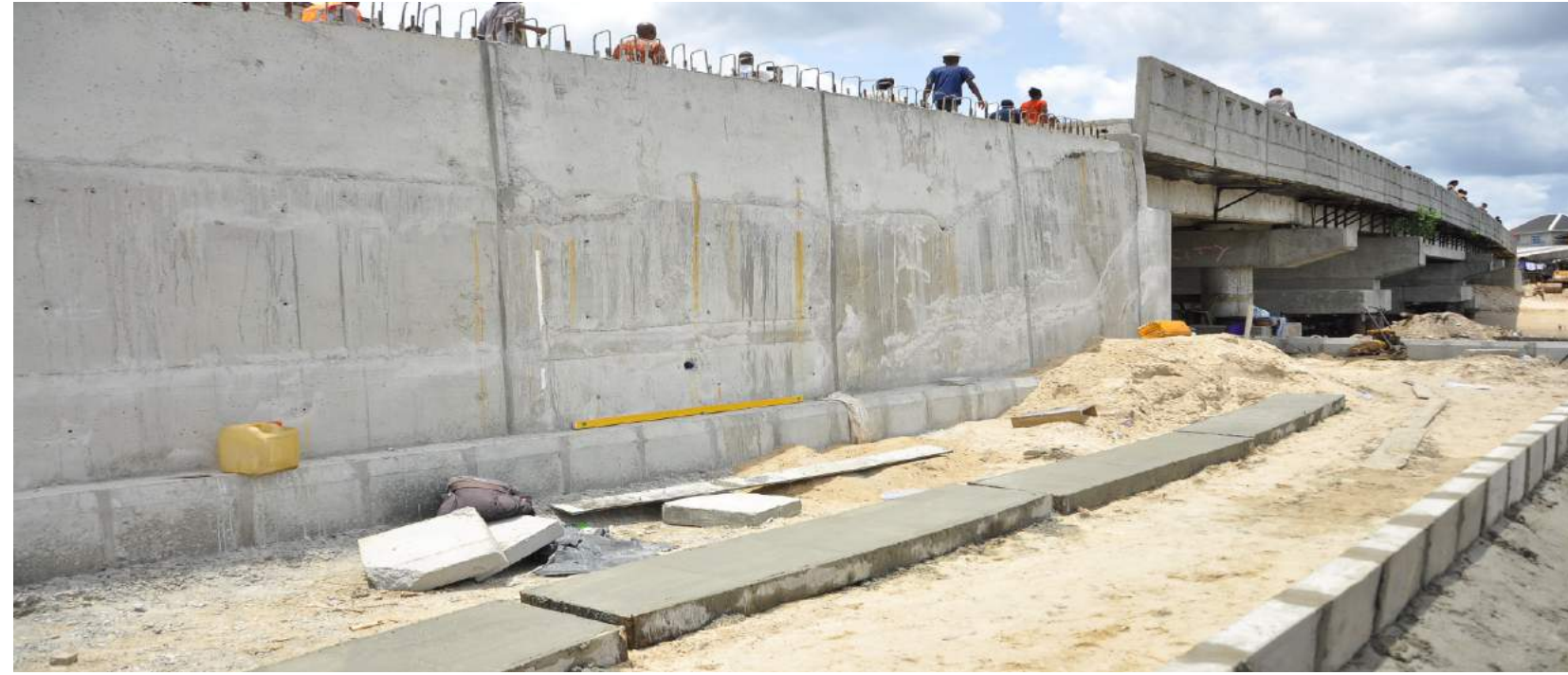
NEMBE UNITY BRIDGE 2 ON-GOING
