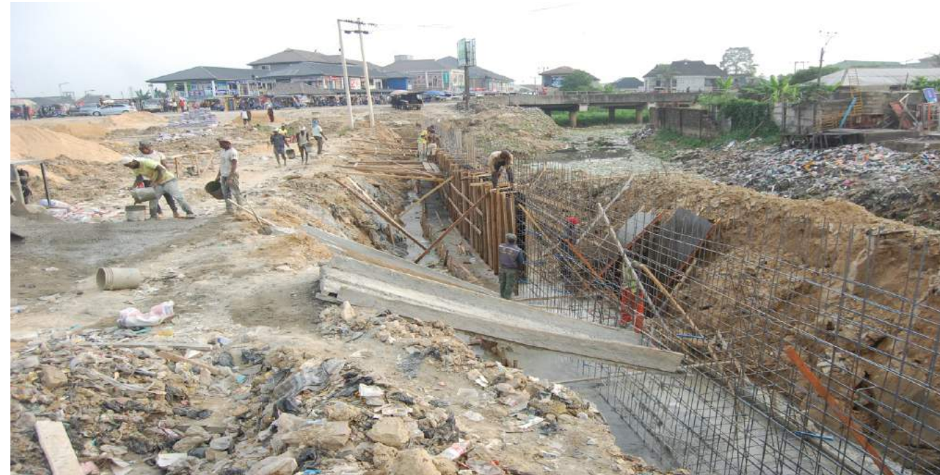
TOMBIA ROUNDABOUT EXPANSION BEAUTIFICATION ON-GOING
