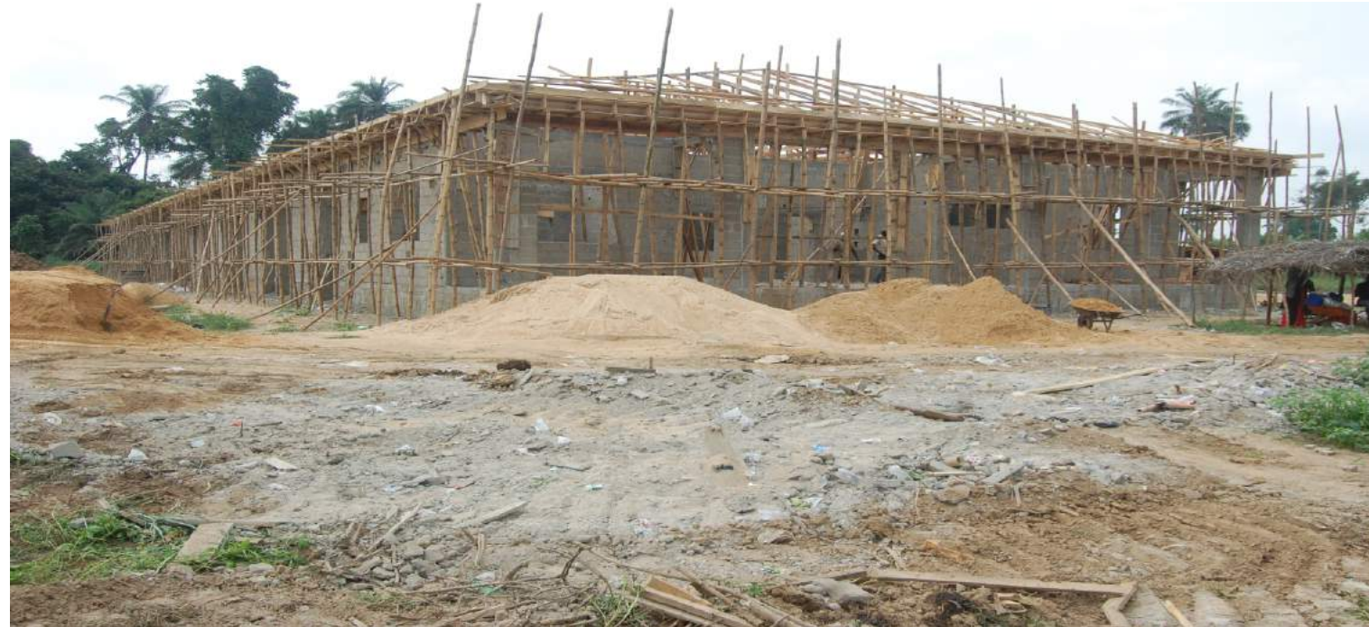
VOCATIONAL CENTRE SAMPOU ON-GOING
