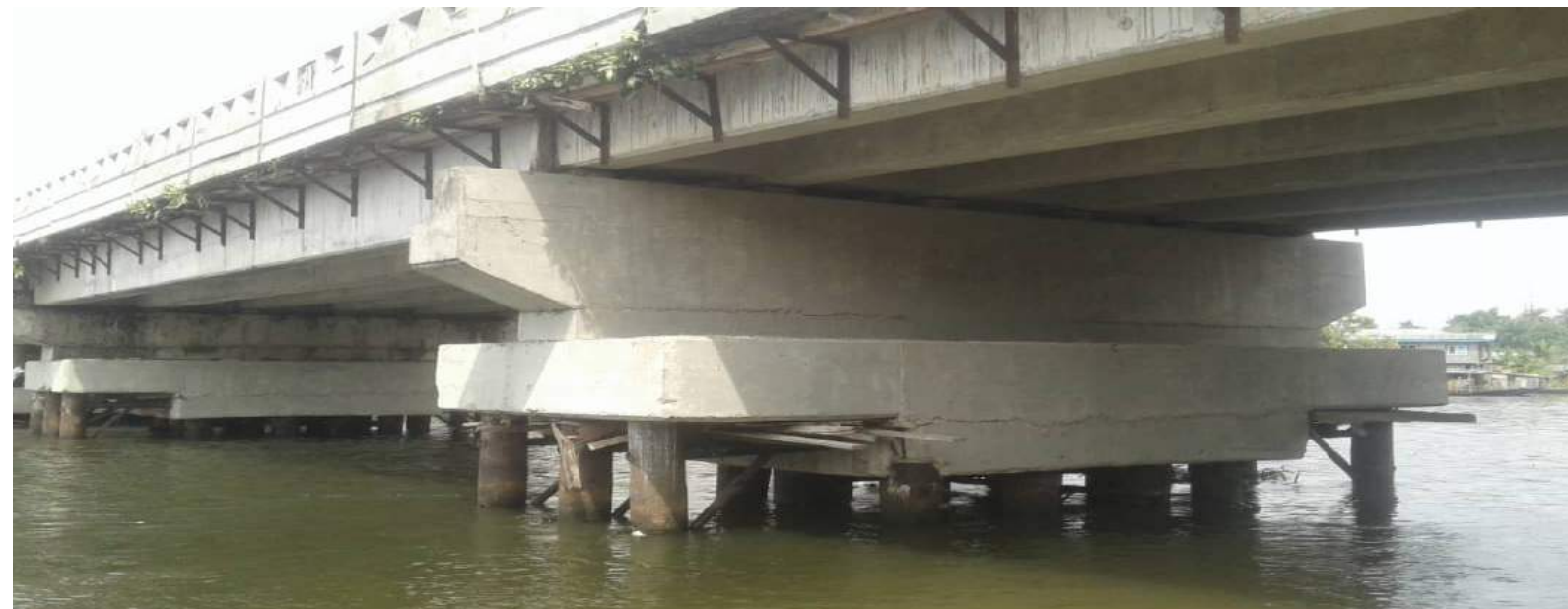
NEMBE UNITY BRIDGE 2 ON-GOING
