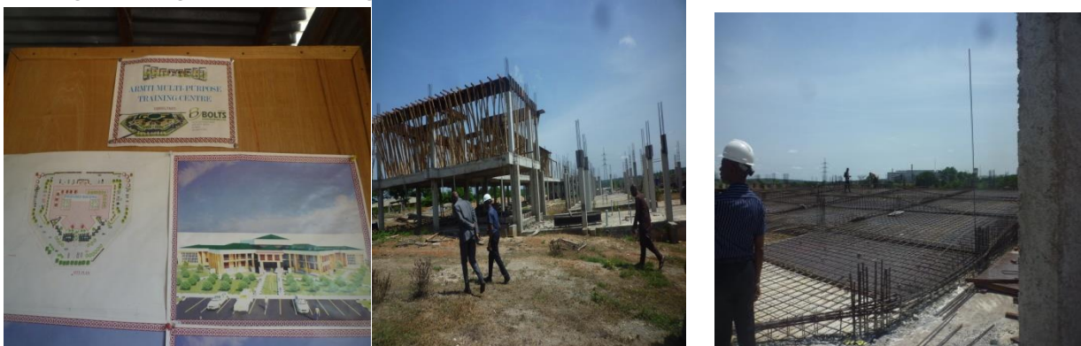
Picture 25: The Ongoing Construction of Multipurpose Training Centre at ARMTI
