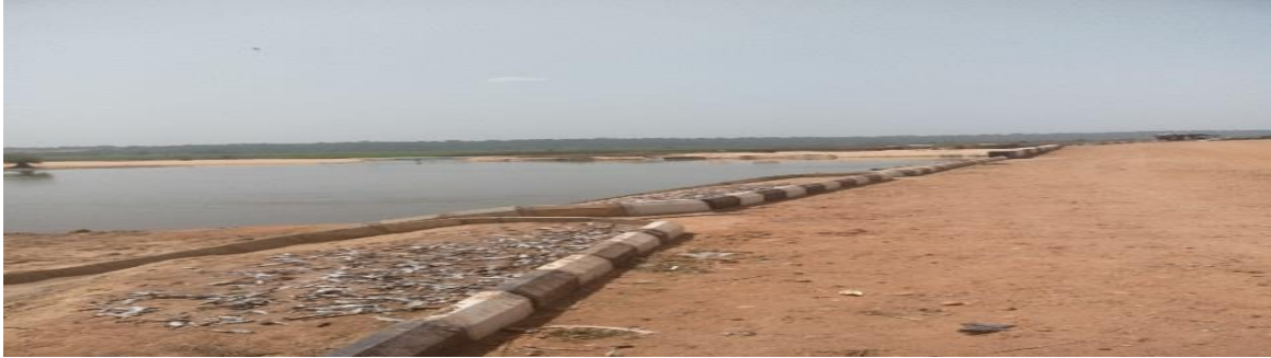
Picture 23: The Completed Embankment (dyke) and Access Road at Tada-Shonga Irrigation Project
