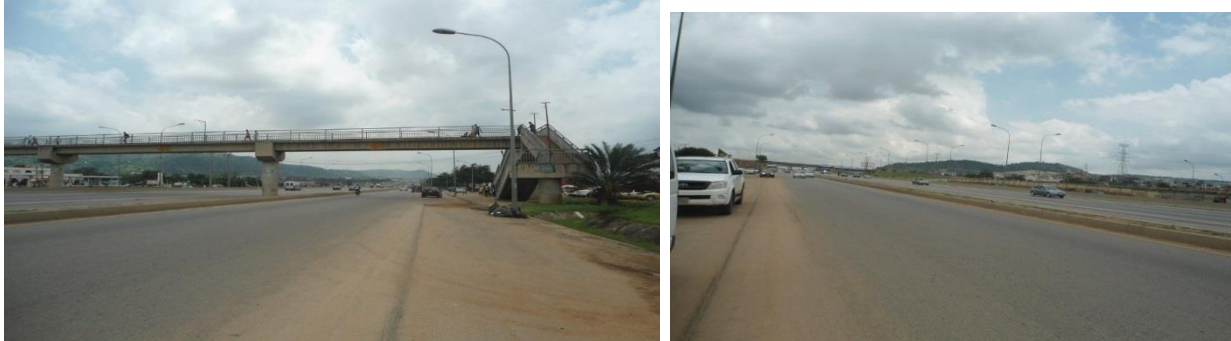
Picture 19: A Portion of the Completed Rehabilitated / Expanded Outer Northern Expressway (ONEX) Lot II
