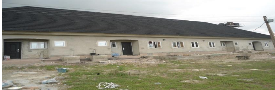
Picture 46: Construction of Hostel at Nigeria Maritime University, Okerenkoko
