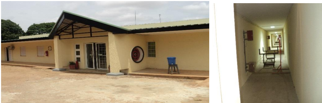
Picture 2: The Rehabilitated Indoor Shooting Range at DICON, Kaduna
