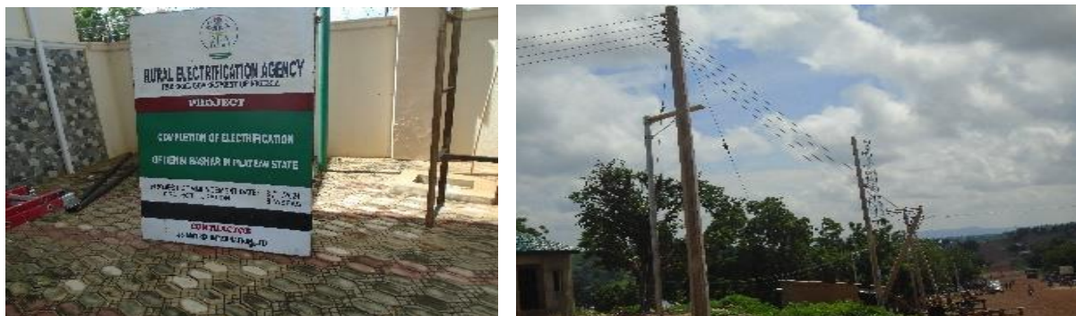
Picture 70: Completion of Electrification of Dengi – Bashar in Plateau, Jos
