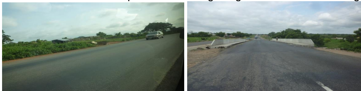
Picture 13: A Portion of Completed Road and Reconstructed Bridge at Bode-Saadu Town of Ilorin-Jebba Road
