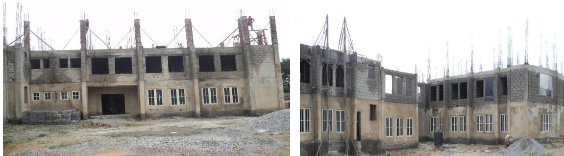
Picture 60: The On-going Administrative Building at the NBTI Headquarters, Abuja
