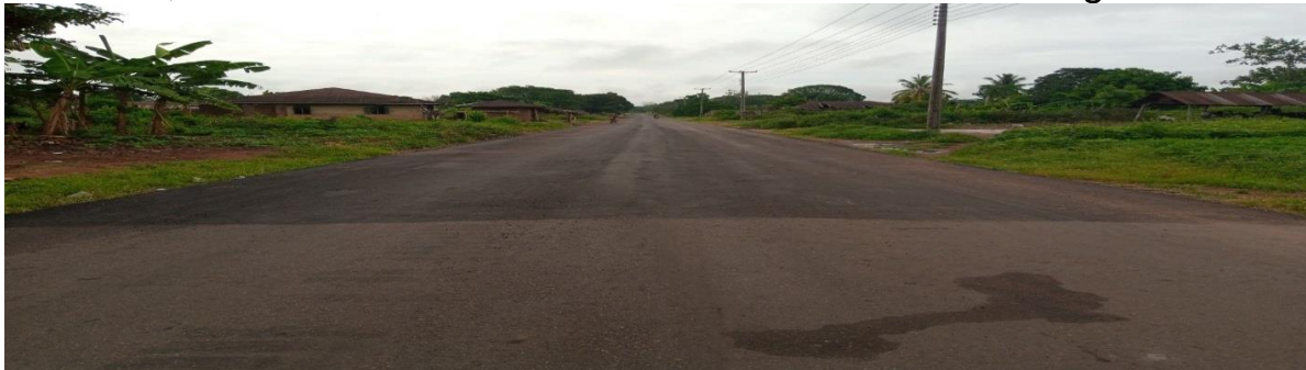
Picture 31: Completed Portion of Ndemili -Utagba-Uno/Ike Road in Delta-State
