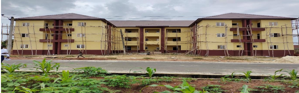
Picture 35: Completed 2 Storey House Officers Quarters.
