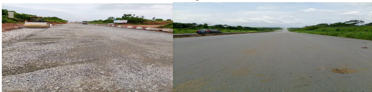
Picture 15: Stone Base Laying Under Progress
