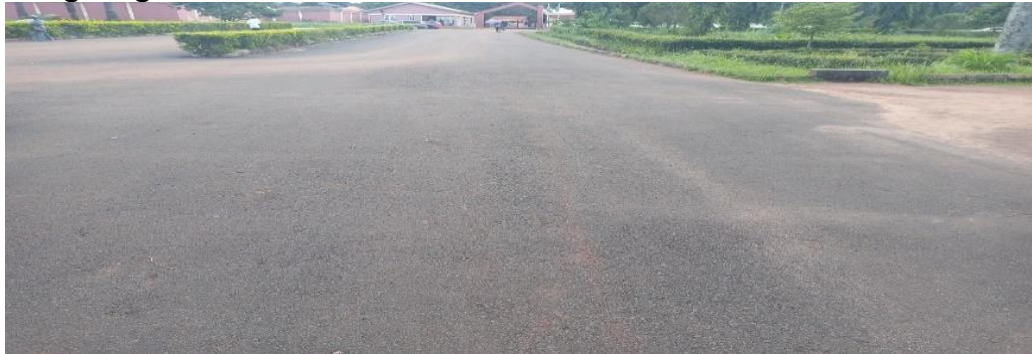
Picture 57: Rehabilitated Internal Road Network at SEDI, Enugu
