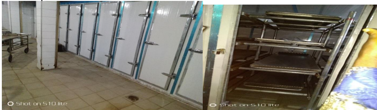
Picture 34: New Fabricated and Installed Morgues
