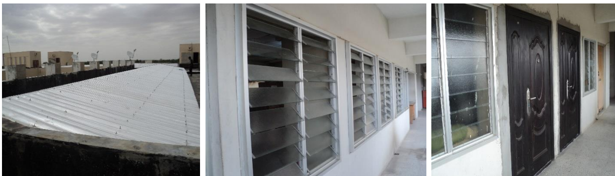
Picture 16: Ongoing Rehabilitation of Federal Secretariat, Maiduguri, Borno – State
