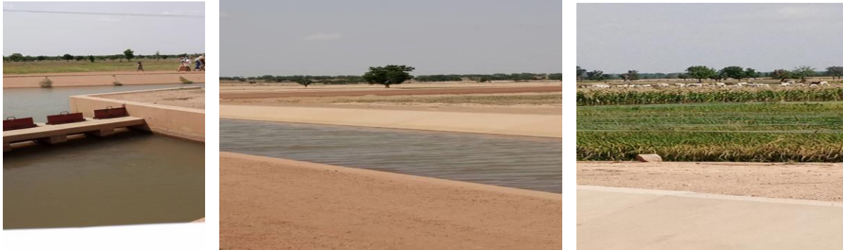
Picture 24: The Spill Way & Completed Sector 4 which was ready for handing over to farmers at the Gari Irrigation Project
