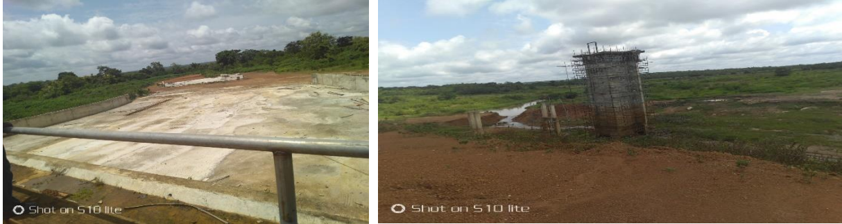
Picture 20: Completed Spillway and Intake Tower at Irawo Earth Dam
