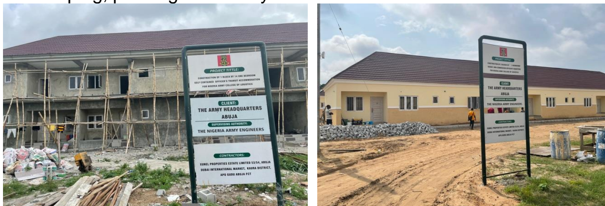
Picture 5: Ongoing Construction of Students Hostel and 2-Blocks of Flats for SNCO at Nigeria Army School of Logistis, Ojo, Lagos State
