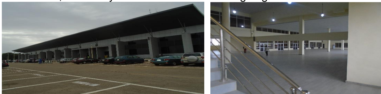
Picture 67: Upgrade and Rehabilitation of Jos Airport Terminal Building
