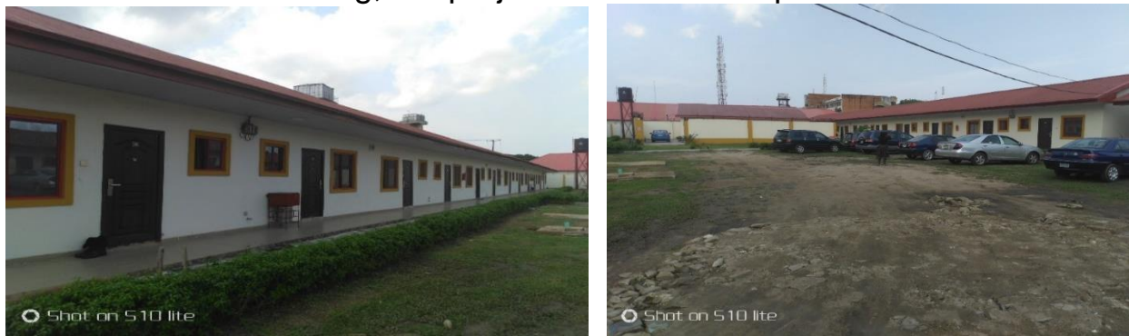
Picture 6: The Completed 36-Rooms Corporal Below Quarters
