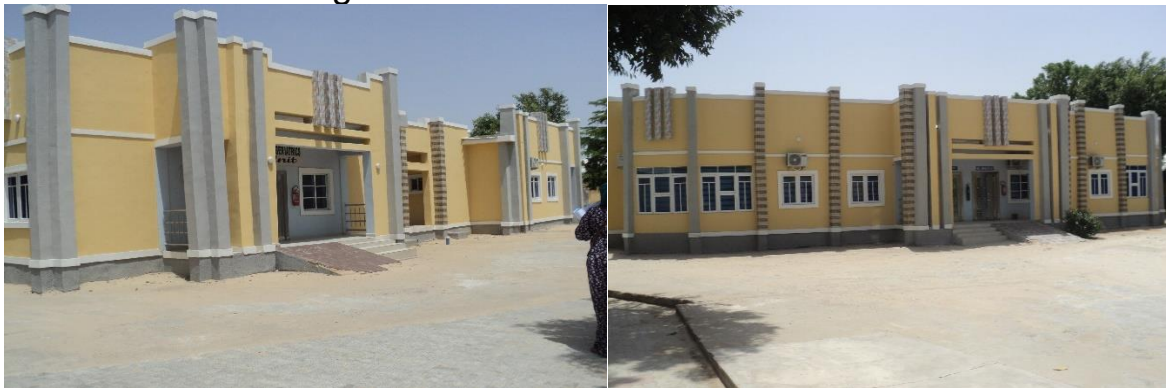
Picture 39: Completed Side and Front View of Psycho-Geriatrics Childrens Complex at the Federal Neuro Psychiatric Hospital (FNPH), Maiduguri
