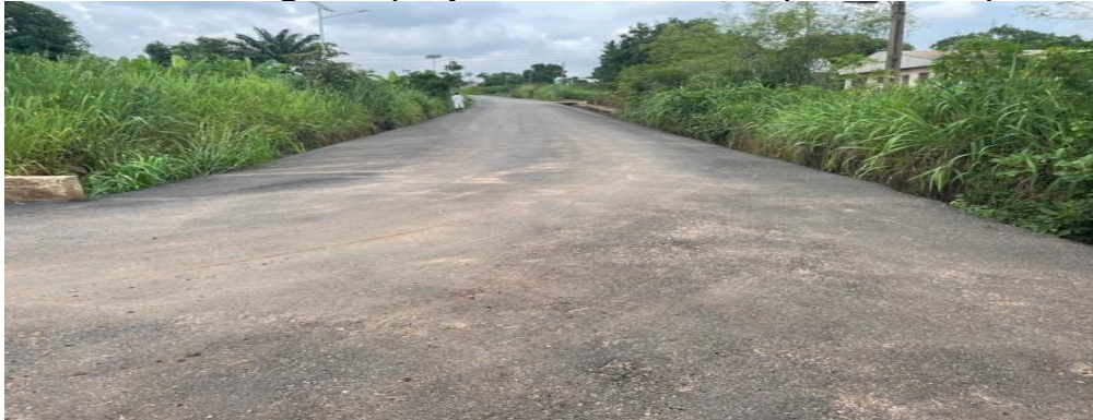
Picture 74: Rehabilitation of Erosion Ravaged Internal Road Phase II
