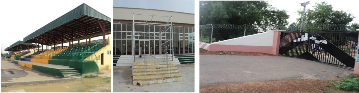
Picture 33: Completed Cross Section of Presidential & Spectators' Pavilions and Fencing at Nigeria Police Academy, Wudil – Kano
