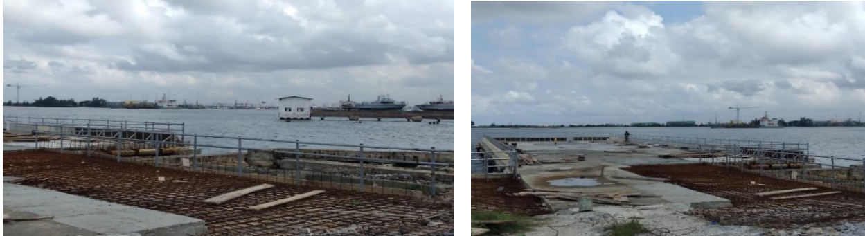
Picture 28: Repairs and Rehabilitation of Jetty and Marine Facility
