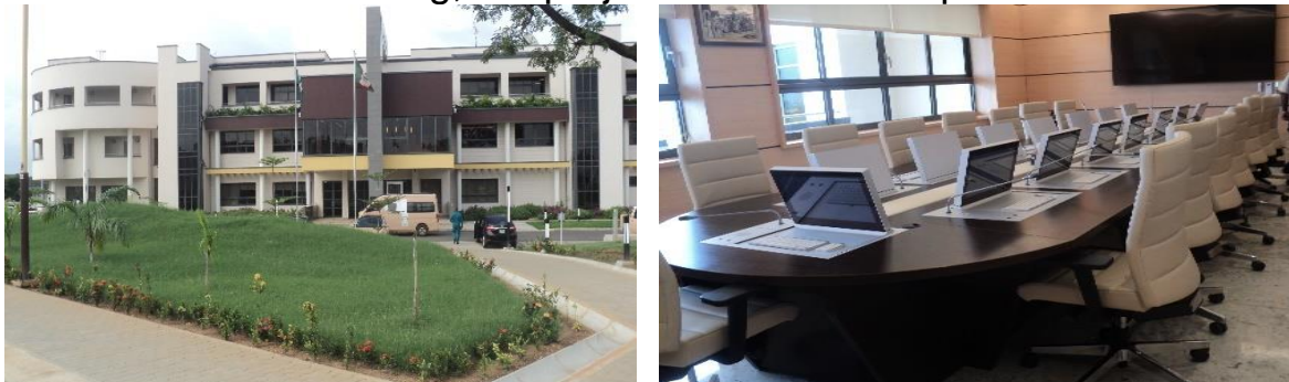
Picture 52: Construction of Technology Building at Nigerian Immigration Service (NIS) Headquarter, Abuja
