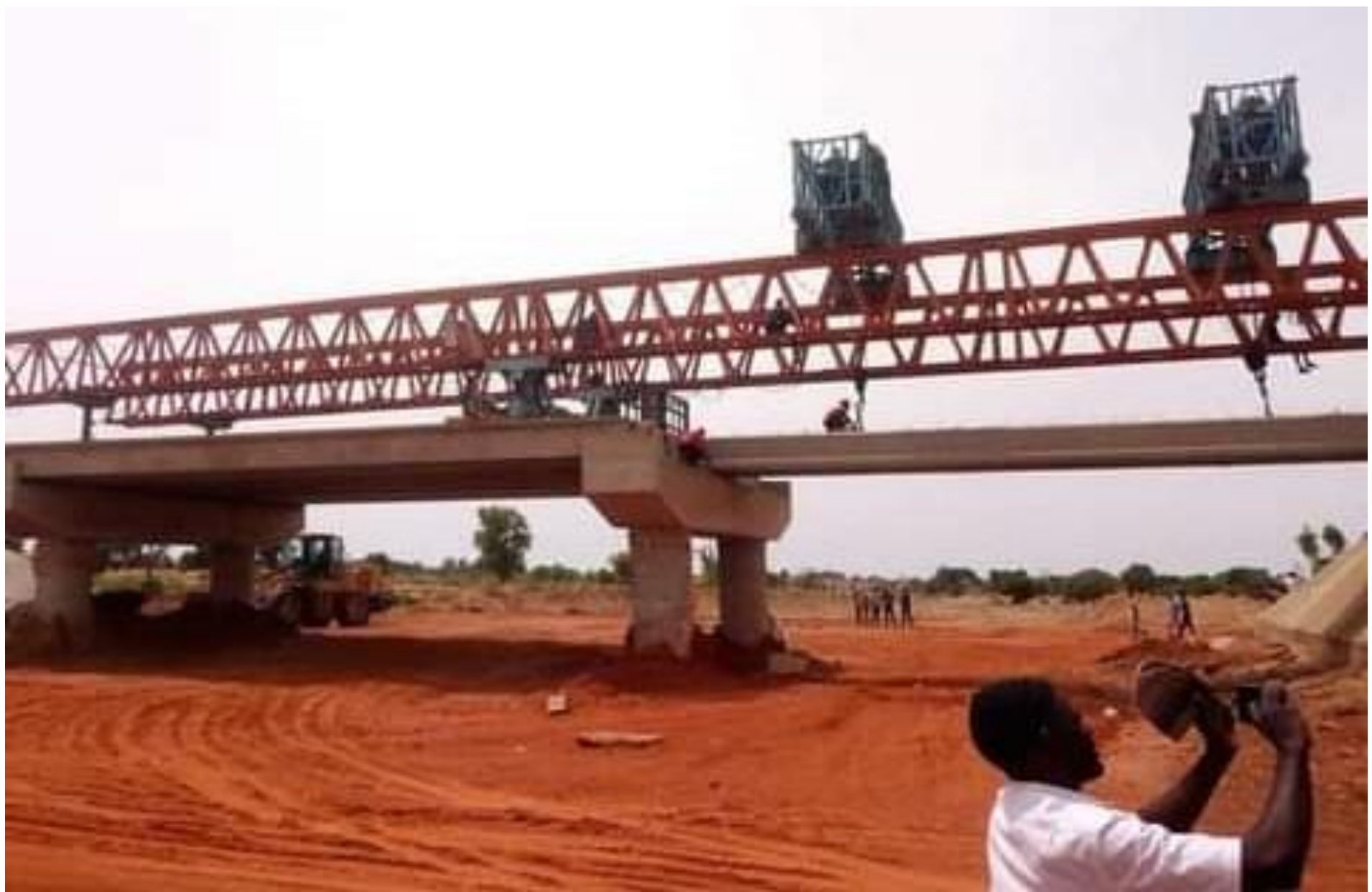
Bapparu Bridge linking Funakaye – Dukku LGA
