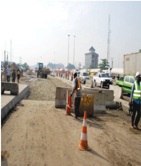
■ Road Rehabilitation work in progress
