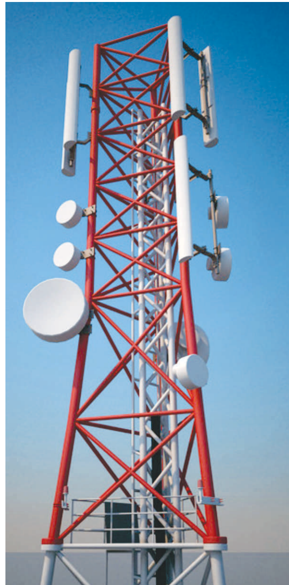
■ Communication Mast in Nigeria
