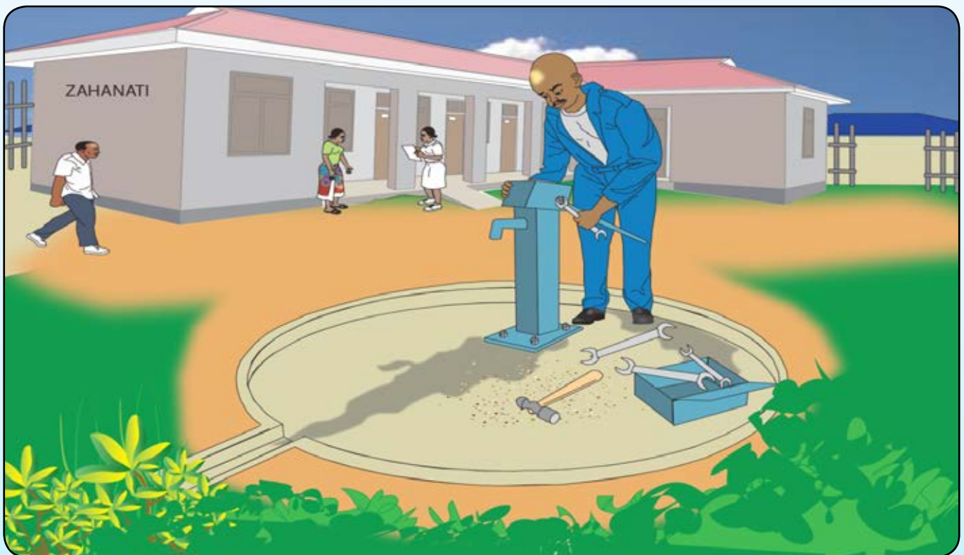
Figure 5.3: Routine maintenance of a protected shallow well fitted in hand pump
