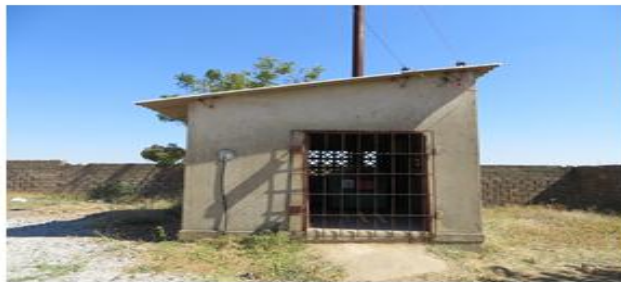
Macro burn incinerator at Monze Hosp.
