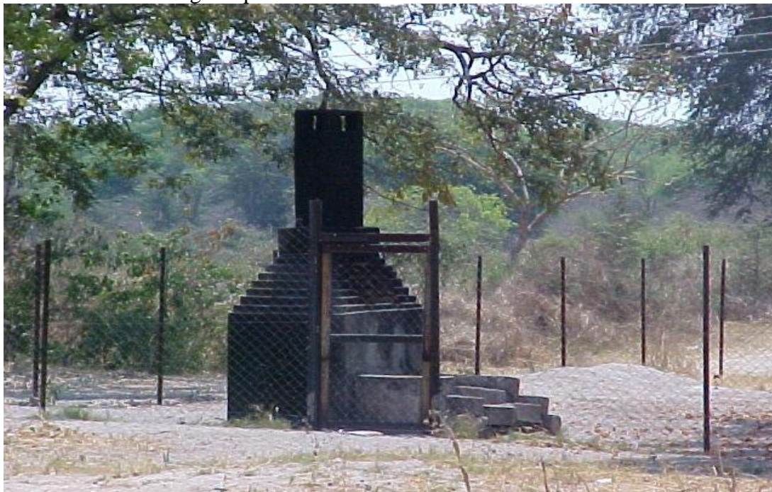
Brick incinerator (Source: ECZ, 2005)
