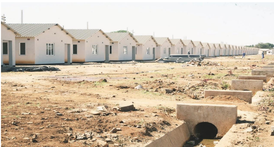
Housing Units under construction by the NBS in Dzivarasekwa
