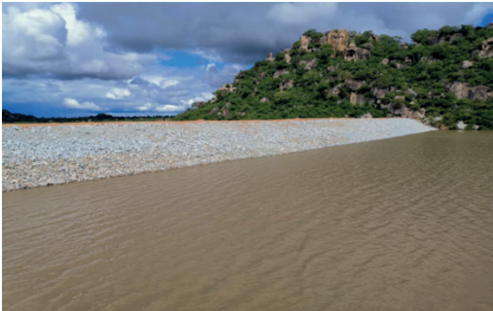
Marovanyati Dam Wall
