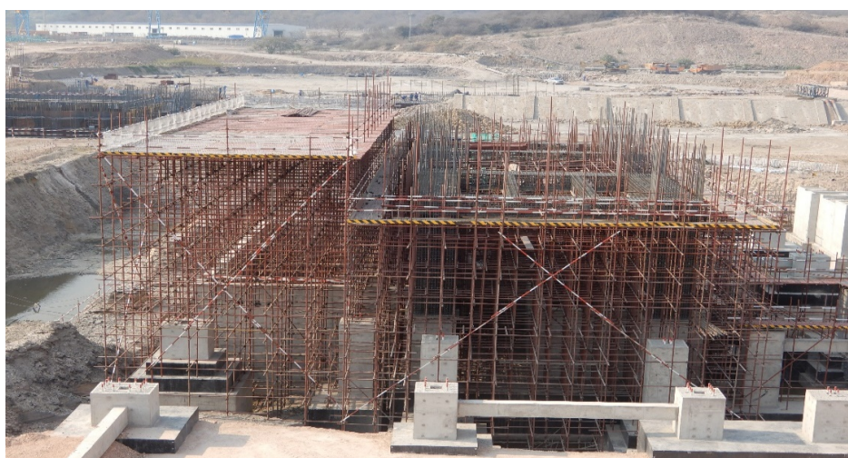
Foundation Works on No. 8 Turbine
