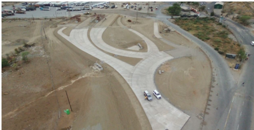
Beitbridge Border Post access area construction.
