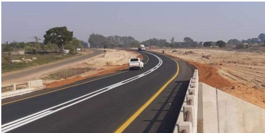
Completed Works on Pembi Bridge, Mashonaland Central
